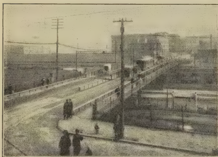
OLD GAY STREET VIADUCT
